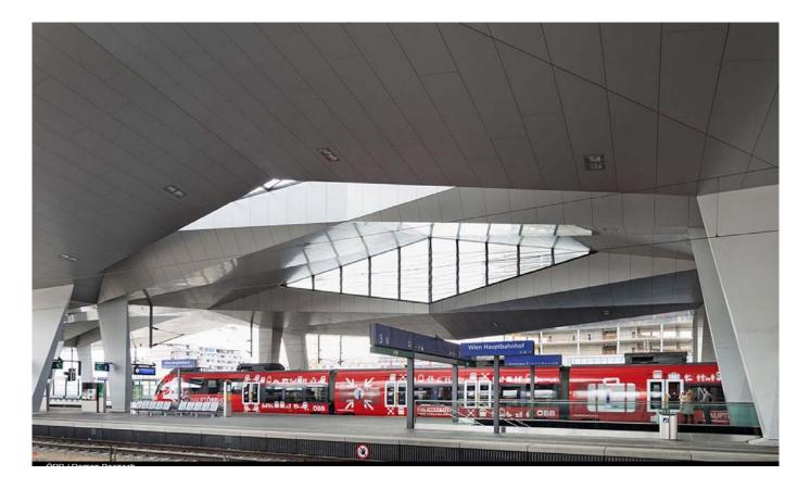
The canopy comprises 14 diamond-shaped space frames, arranged in five rows that follow the lines of the tracks and each of the platforms.
